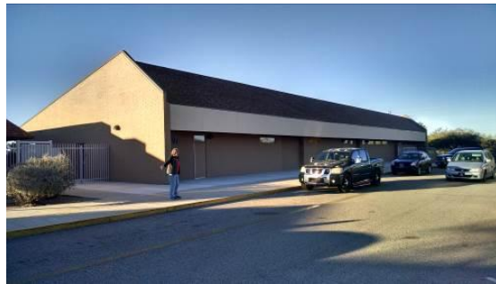
North Face of New Building
