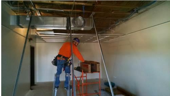
Building W2 Renovation
