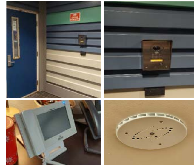
Clockwise from top left: Tikiġaq site entrance cameras, office video/audio door release, vape detectors
