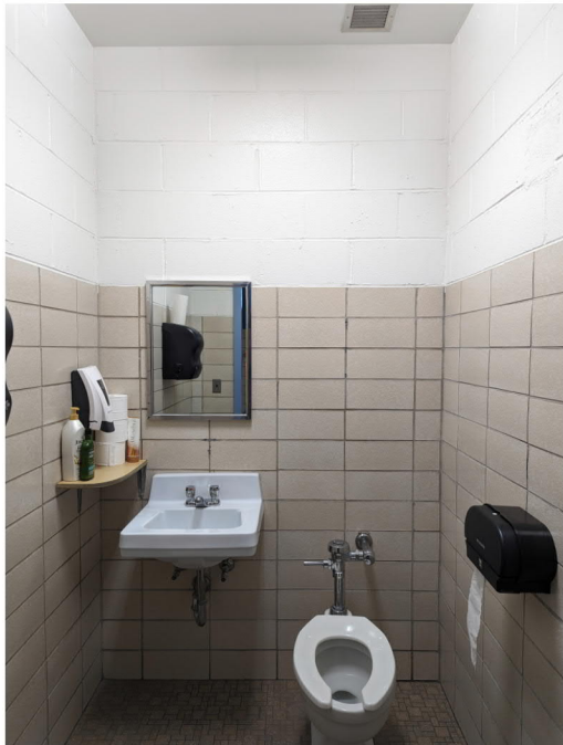
SECOND FLOOR STAFF TOILET (T3)
