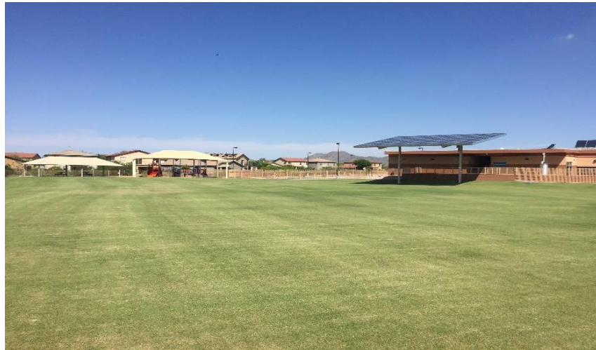
Solar Array and Canopy's
