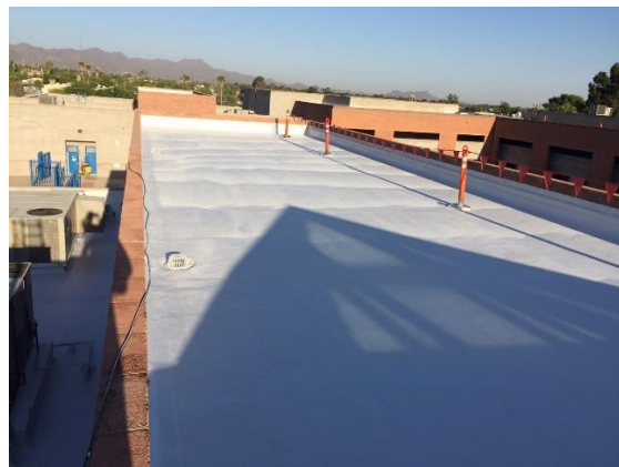
Keeling Administration Roof
