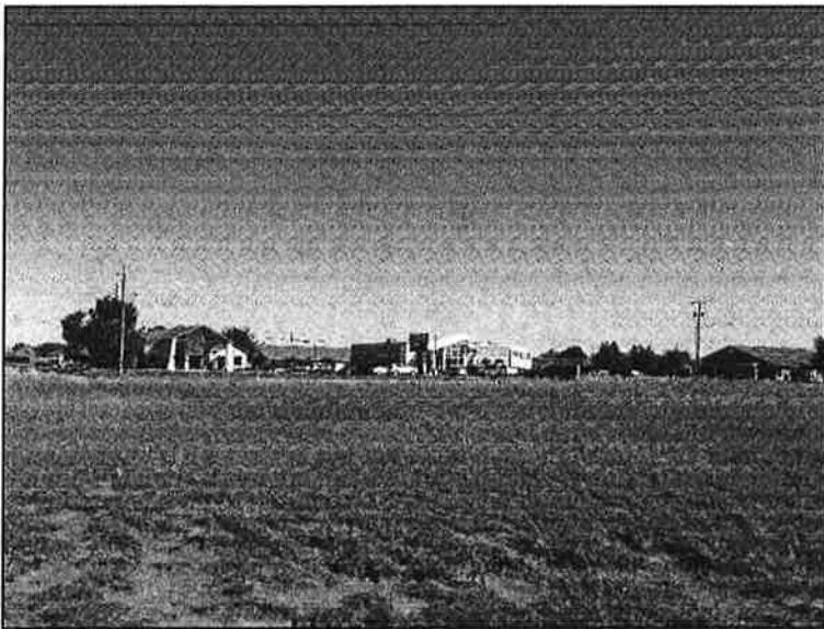
2675 Northwest Loop Overall View of Subject Looking Northeast
