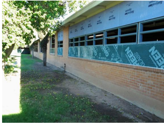
500 Wing Window Replacement
