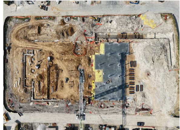
Overview of site – Slab on Grade at start of Concrete Curing
