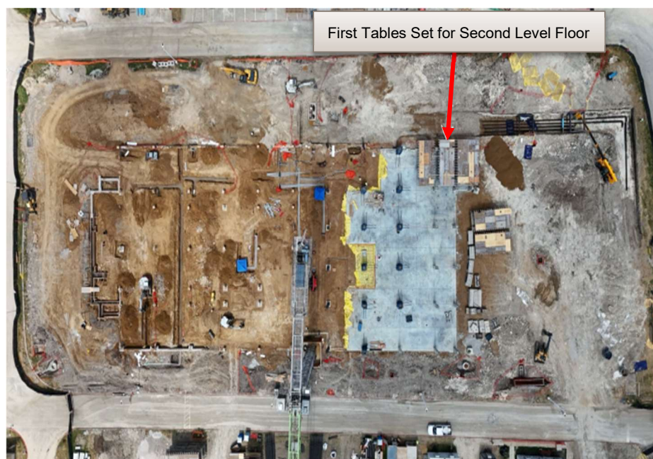
Overview highlighting First Tables Set for 2 nd Floor
