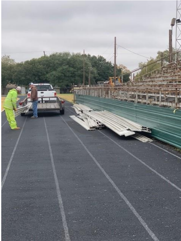
Demolition and Disassembly of Bleachers at Stadium
