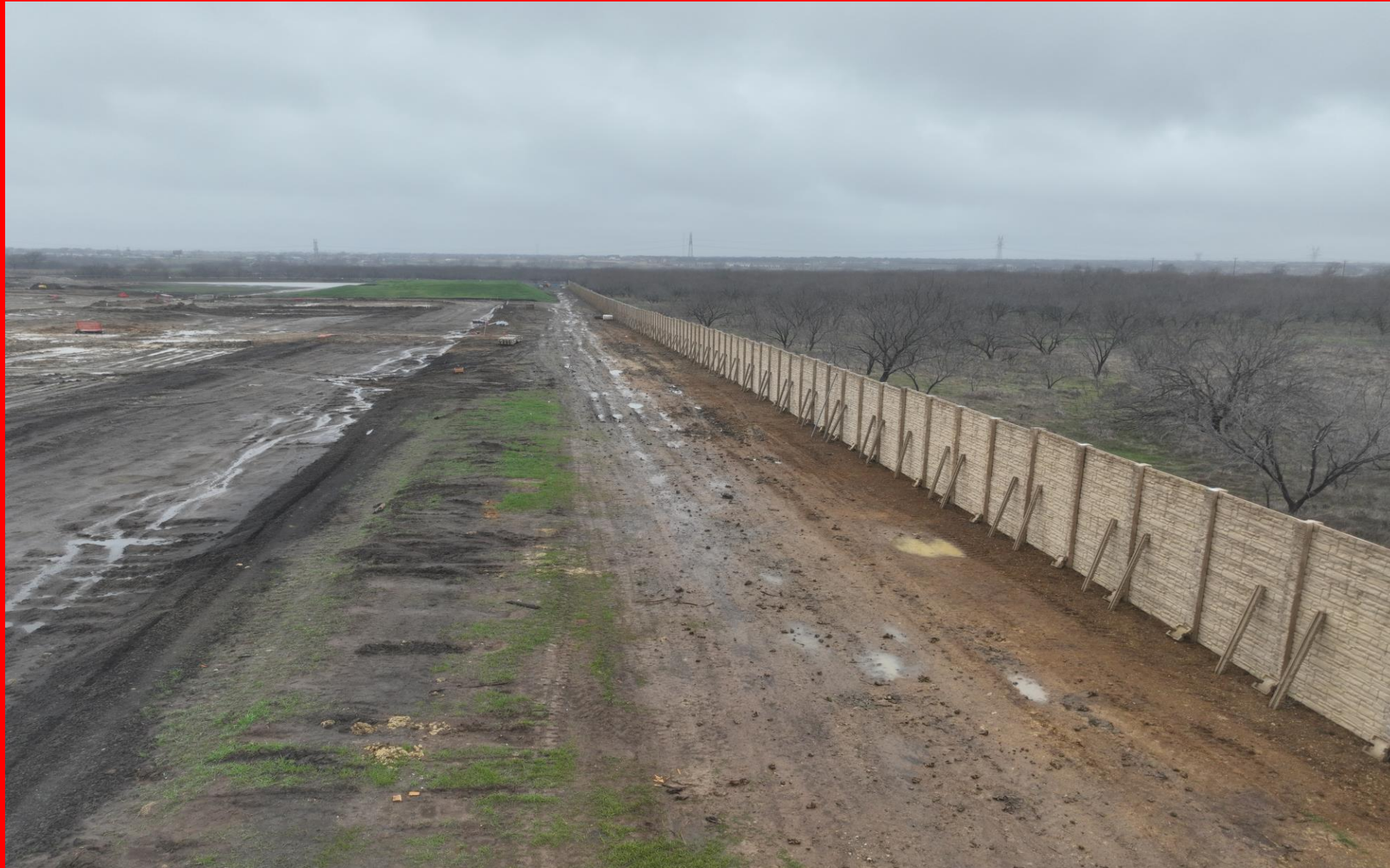
Precast Concrete Fence North Side
