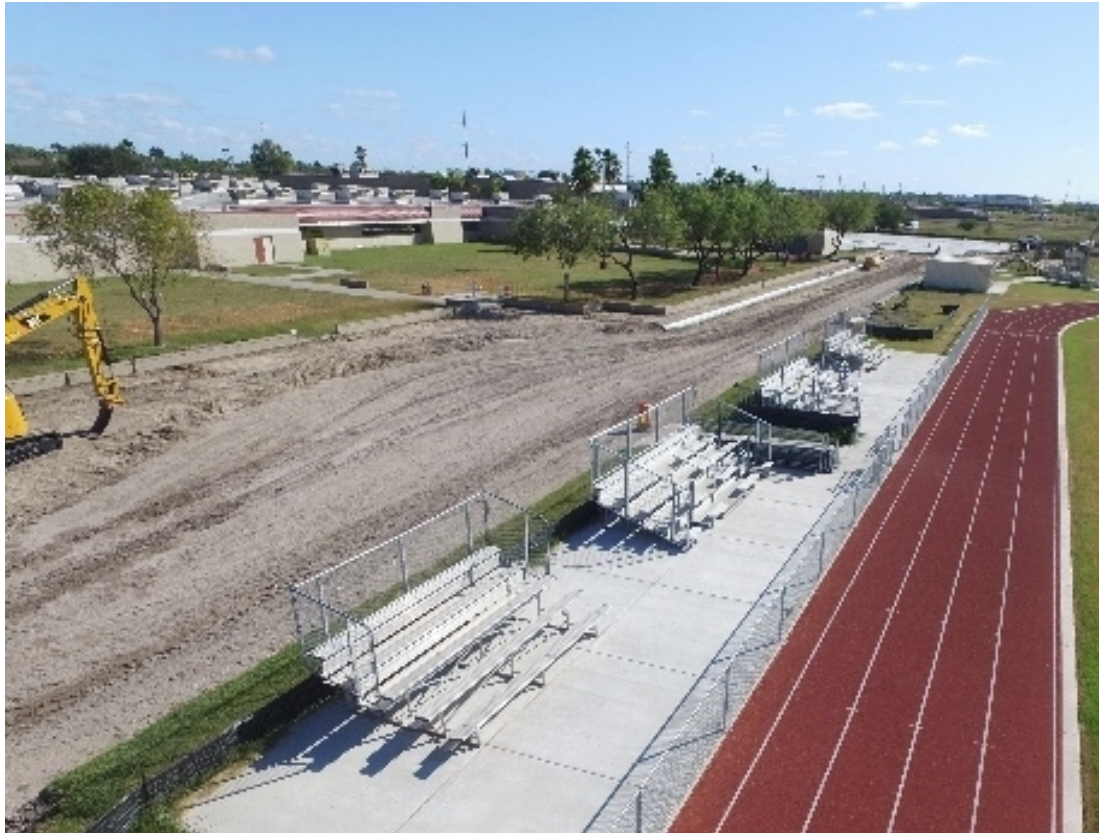
Vela MS -Bus Drive Improvements 40% Complete
