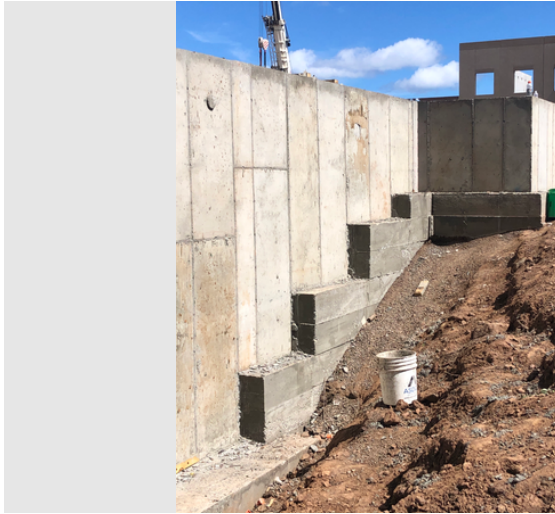
Description Step Footings at Transportation
