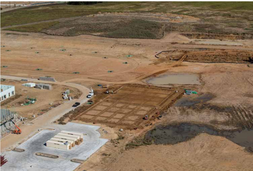
Tennis Court grading and foundation in progress.
