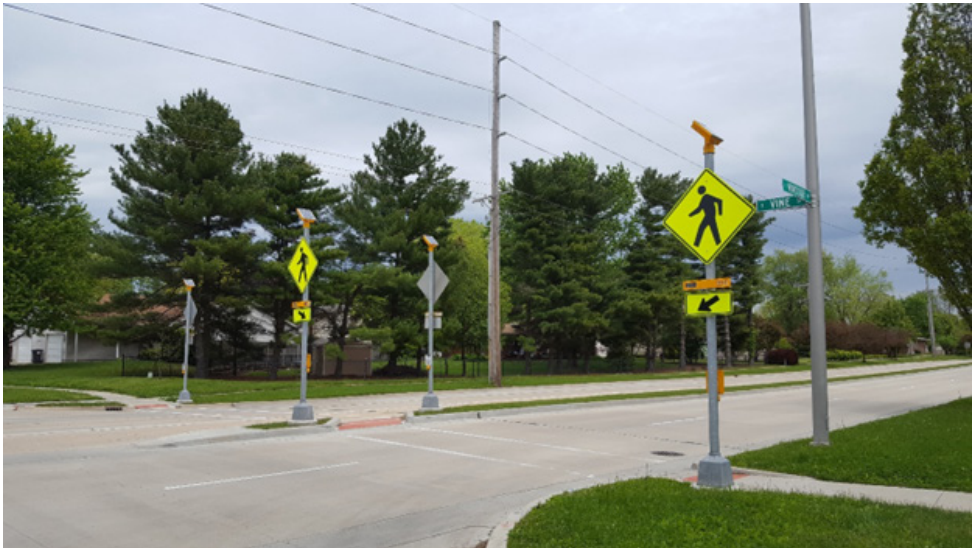
Figure 15: Rectangular Rapid Flashing Beacons (RRFB) and a median refuge island in Urbana
