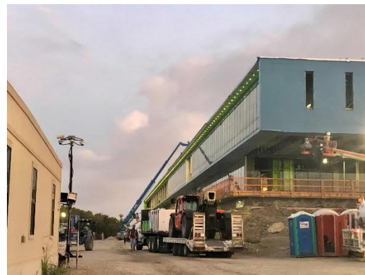
Eyebrow Lights Installed on West Side of the Academic Building
