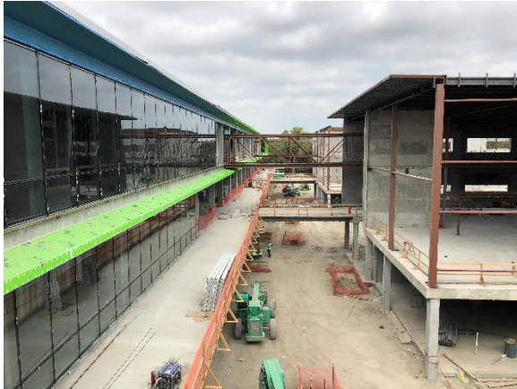
Bioswell, Looking North, from Building A to Building B Bridge
