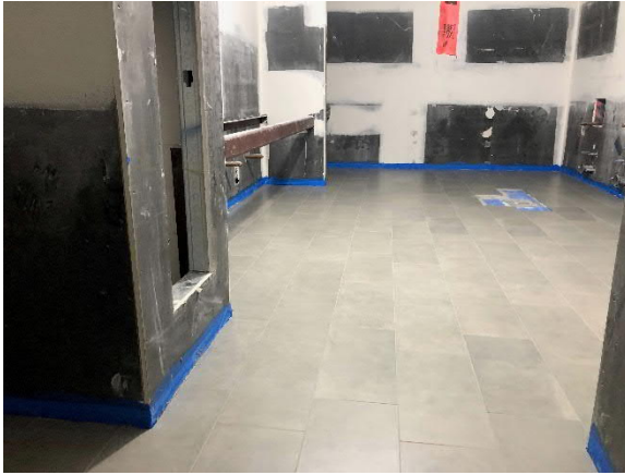
Restroom Tile Install at Library
