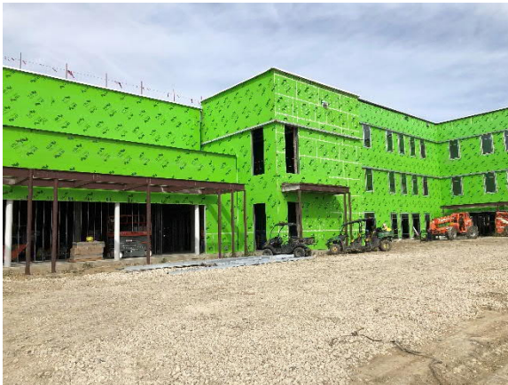
Sheathing on East Side of Conference Center
