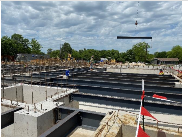
Fig 2: Steel floor framing Area B
