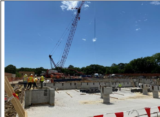
Fig 1: Staging in Area A
