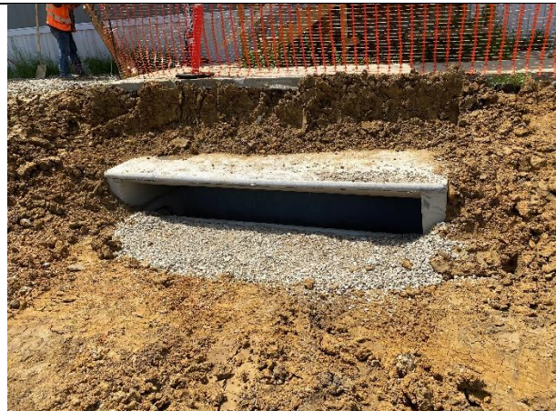
Fig 10: RCP/inlet installation west drive
