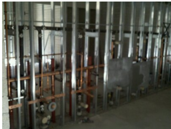
Interior MPE Installation
