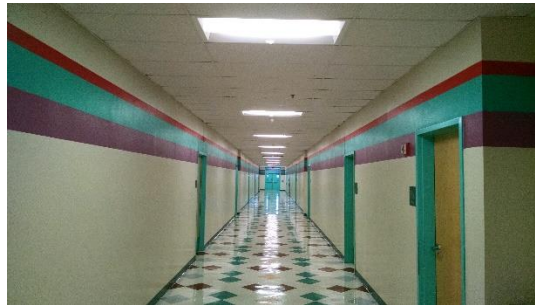
LED Lighting Upgrade
