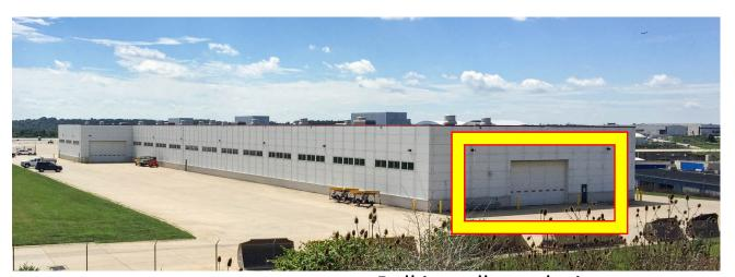
Roll in, roll out design prevents damage to building and doors by eliminating vehicles backing in.
