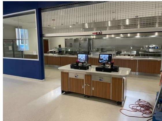
Serving Area in Dining Room
