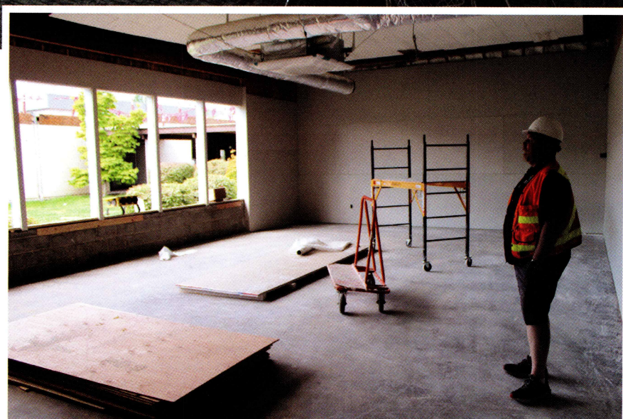
Talent Elementary School classroom during renovation, before and after.
