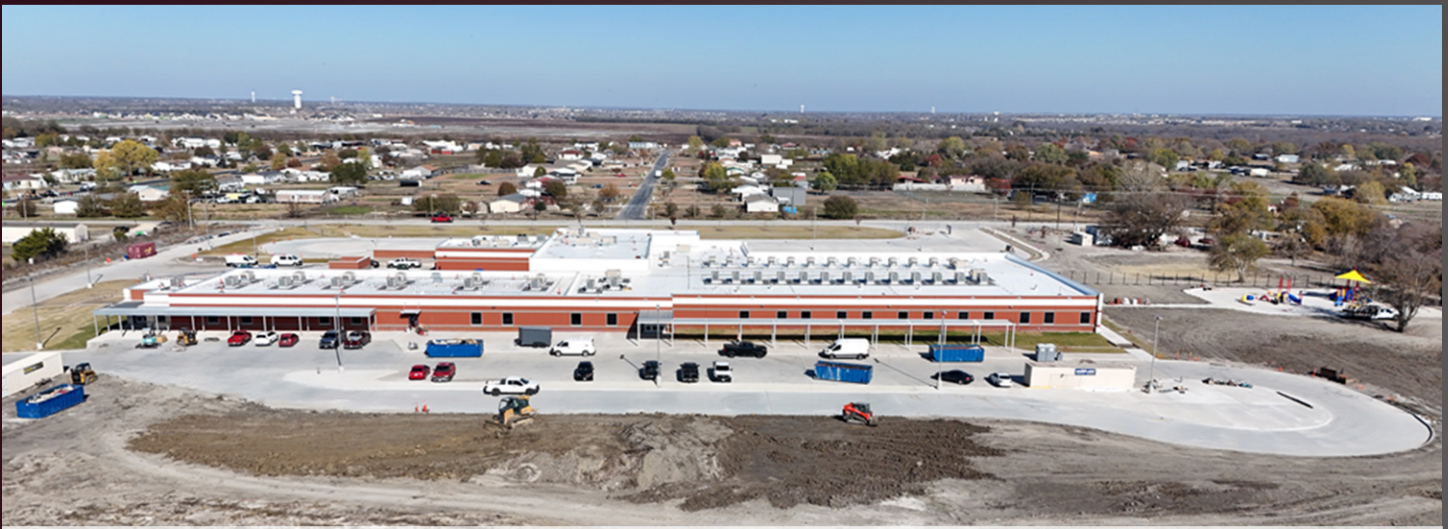
VIEW LOOKING NORTH
