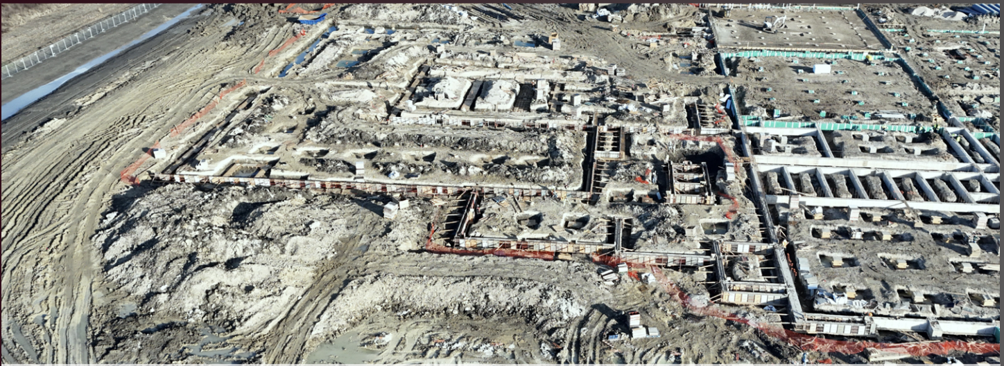
VIEW LOOKING NORTH
