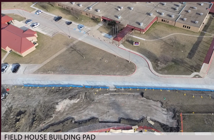
FIELD HOUSE BUILDING PAD
