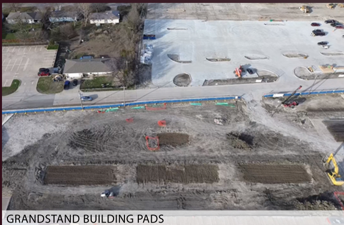
GRANDSTAND BUILDING PADS
