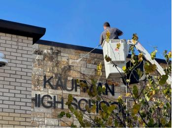
In November, the maintenance crew used a lift and power washer to clean the walls of the high school. This process keeps the building looking new.
