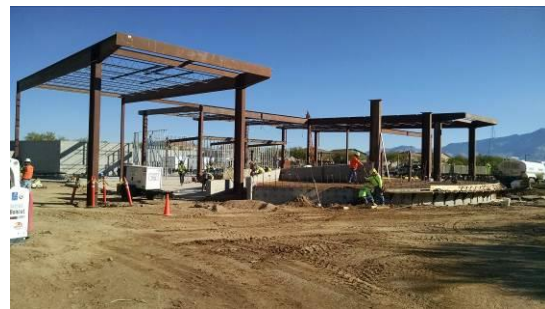
300 Building Stage Before Concrete
