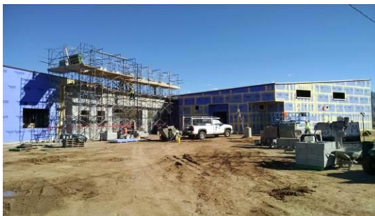
Buildings 100 & 200 in progress
