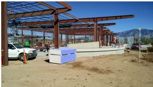
300 Building Stage After Concrete
