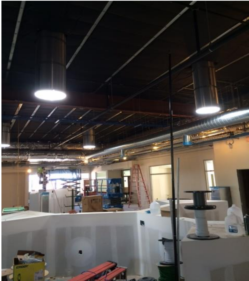
400 Building lighting from windows and skylights only
