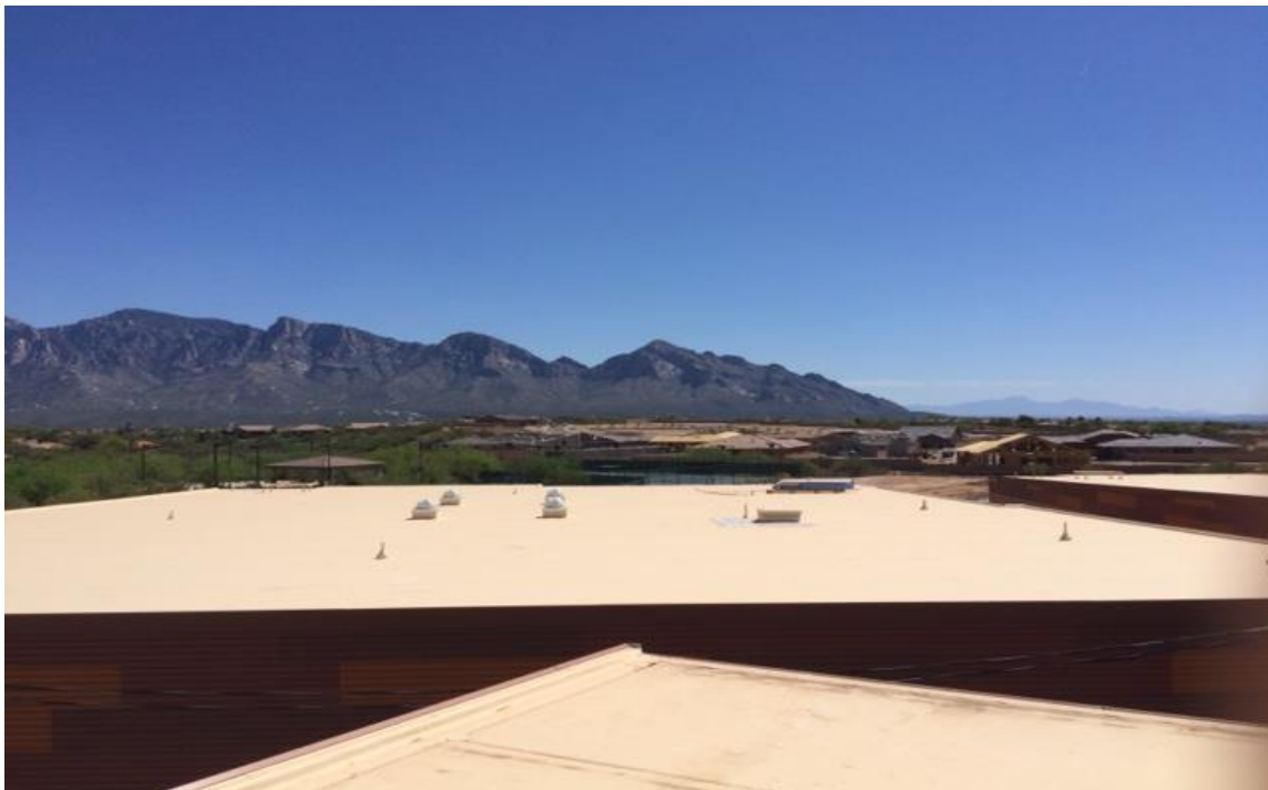
View from Building 300's roof viewing building 400's roof
