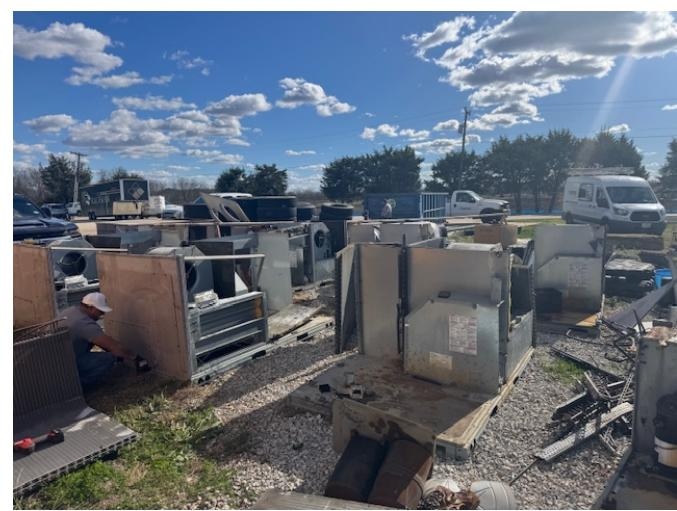
**In January, the crew took some time to break down some old HVAC units so that the parts could be processed. They recovered the refrigerant and recycled the metals.**
