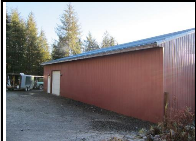
SEISDNBBF Biomass Boiler Facility. Just commissioned a few weeks ago.
