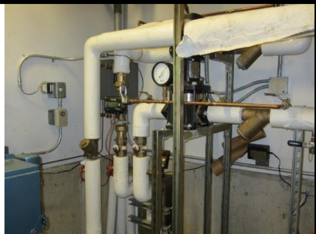
SEISDTBS Biomass heat exchanger. Simple yet very effective.
