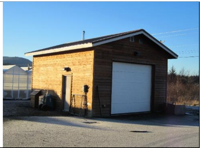
SEISDCCBBF Biomass Boiler Facility.
