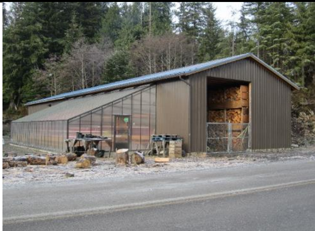
SEISDTBSBBF Front portion of facility is being used to dry wood.
