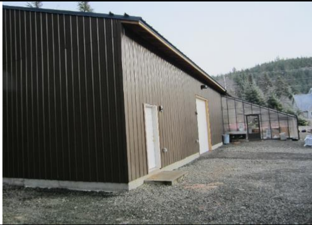
SEISDTBSBBF Greenhouse –right of photo- is partially attached to the boiler facility.
