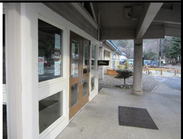
SEISDTBS Main entrance.
