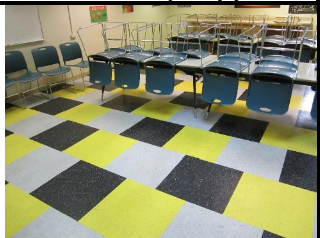
SEISDTBS New tiles. It was mentioned that yellow is one of the toughest colors to keep clean. Currently in great condition.
