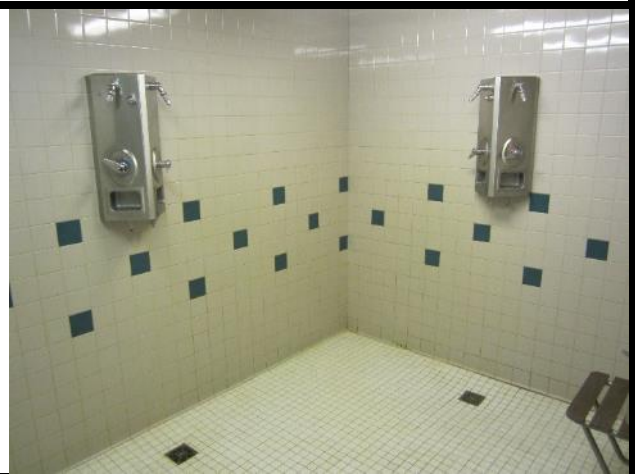
SEISDTBS Shower stalls.
