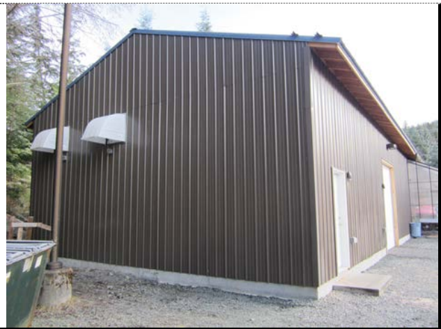
SEISDTBSBBF Biomass Boiler Facility.
