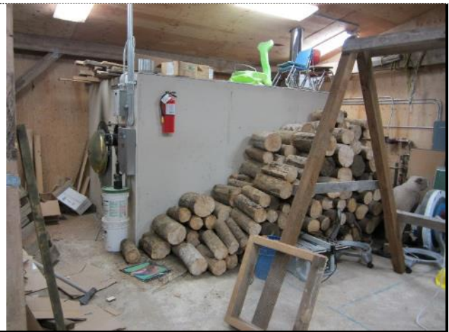
SEISDKBBF Single boiler for small campus.
