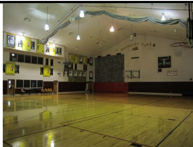
SEISDTBS Lighting upgrade listed priority 6 on CIP list.
