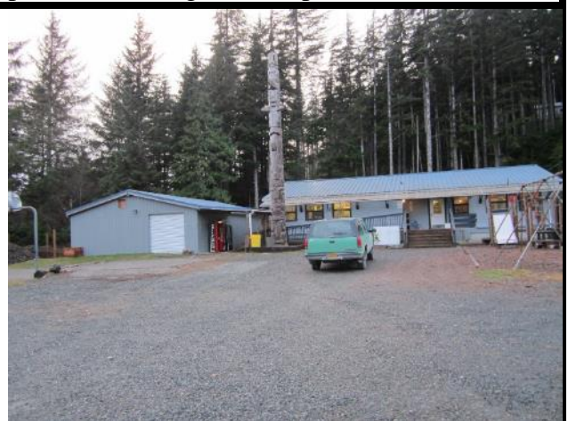
SEISDKBBF Kasaan Biomass Boiler Facility (left). School is to the right.
