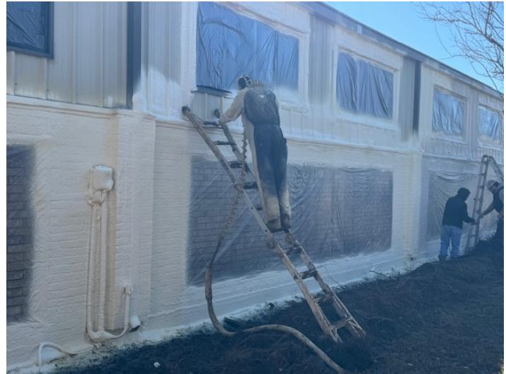
The maintenance crew teamed up with contractors and student workers to add a final coat of foam to seal the gym at Phillips Elementary. This final layer should keep the water from infiltrating that space for years to come.
