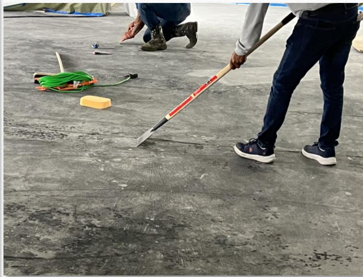
Preparing the floor to seal it.
