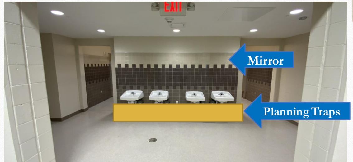
Pending - covers for plumbing traps
