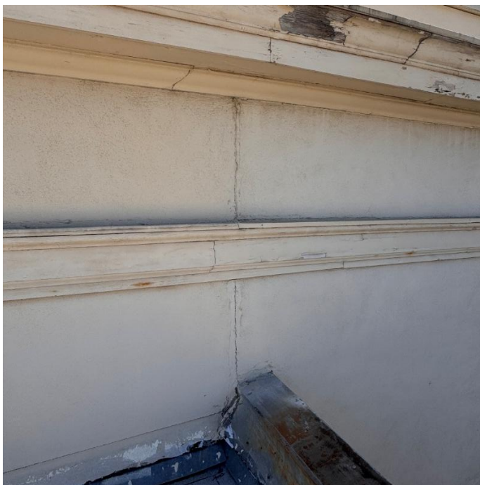
Photo #17. Looking Northwest. Refer Photos #9 and #10. This crack is at a location that is common to buildings indicating expected expansion and contraction.
