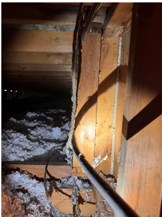
Photo #18. Looking West. This picture indicates a stooled-up frame wall running west the length of the gymnasium. It bears on the ceiling framing and continues up underneath the roof framing.
