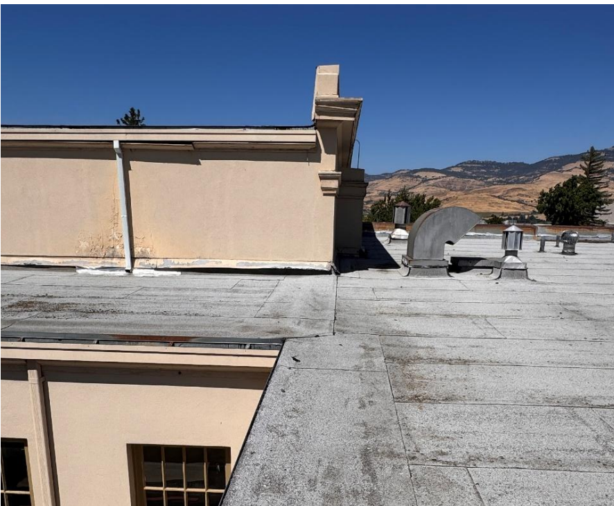
Photo #16. Looking North. Refer to Photos #9 and #10. Note the hump from this lower eave to the corner of the gym indicating movement. The buckle is directly below the corner of the gym.
