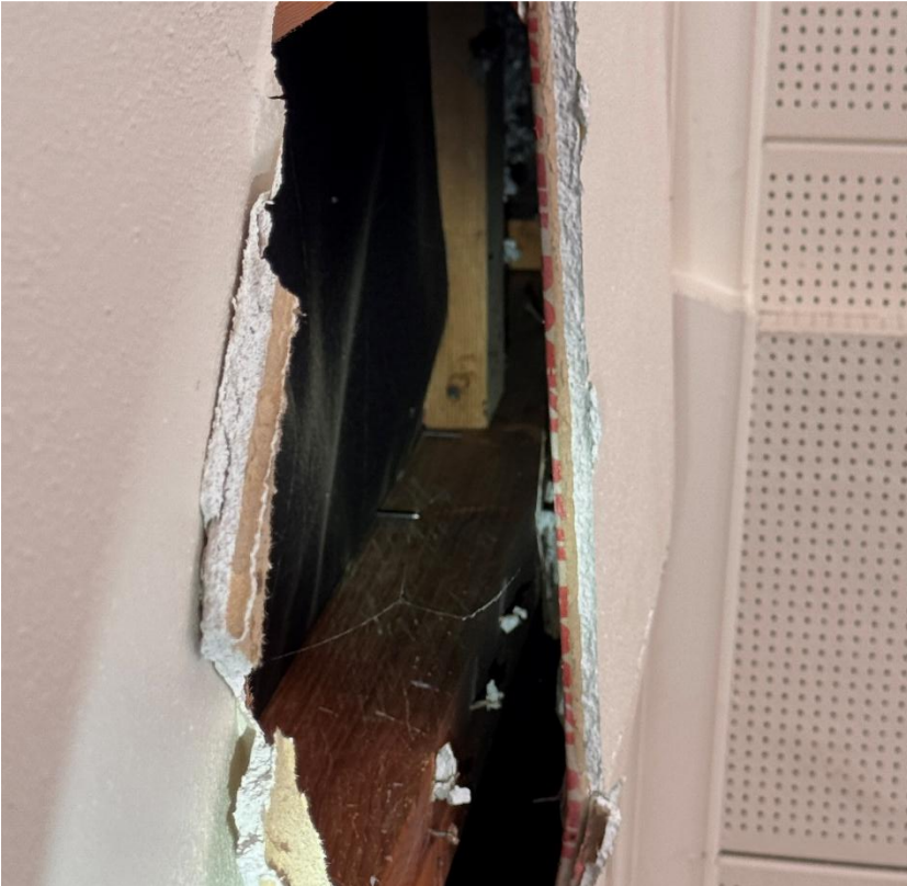
Photo #13 Looking Northeast. Refer to note #10 above. This recent framing is intriguing as it may indicate an intentional repair near the ceiling level.
