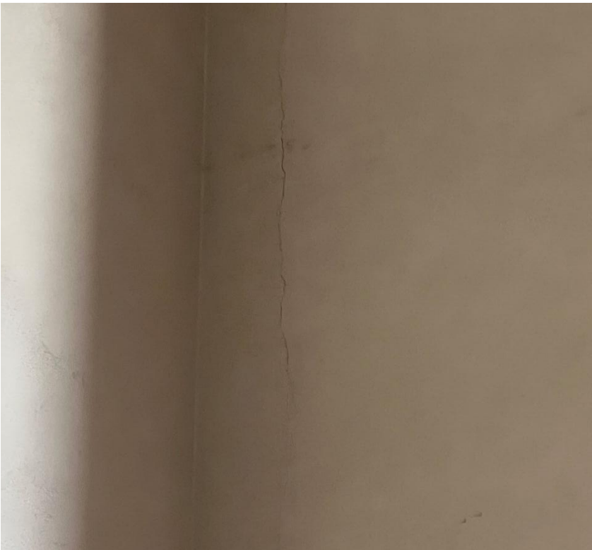
Photo #5 Looking west. This shows a plaster crack indicating minimal building movement.
