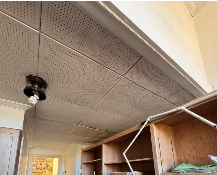
Photo #14 Looking Southwest. The buckle is on the outside of this wall. The water stains at acoustic ceiling may indicate water from outside or from the HVAC equipment in the mezzanine above.
