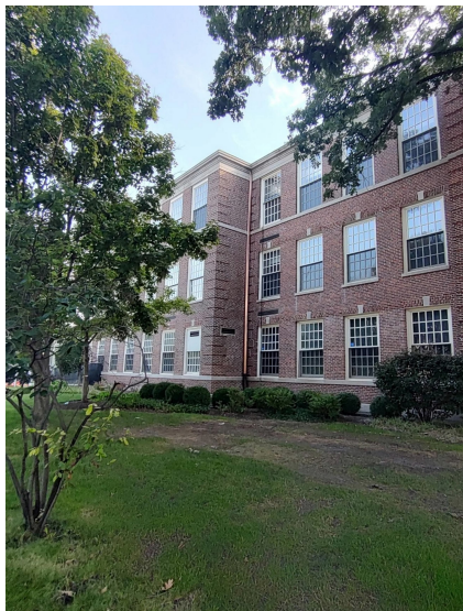
DOWNSPOUTS IN PLACE
