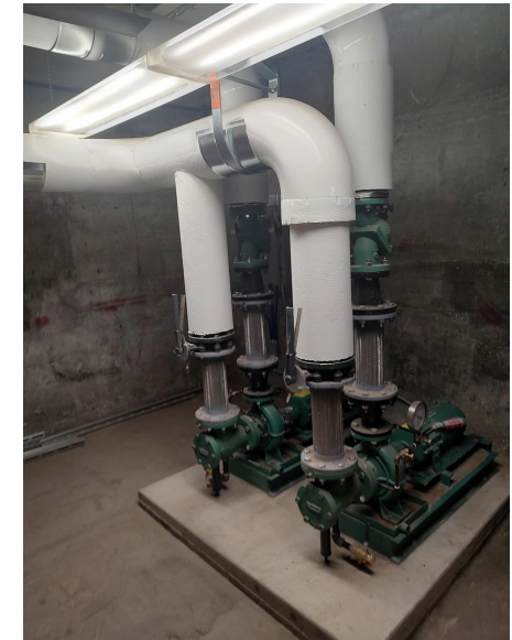
INSULATION WORK COMPLETED
