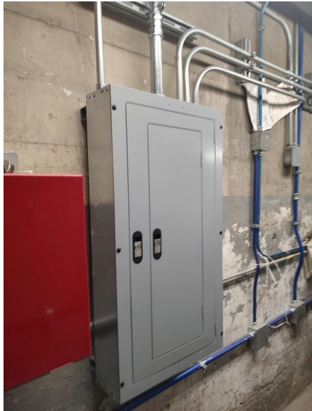
CONTROLS ROUTED AND INSTALLED
