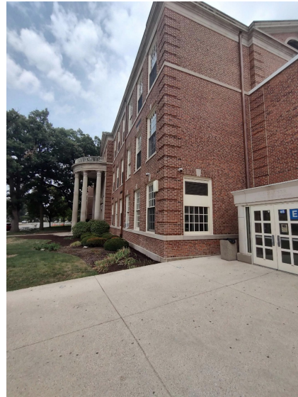
TUCKPOINTING & WASHING COMPLETE
