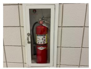
**Photo 188:** Typical portable fire extinguisher in cabinet.
