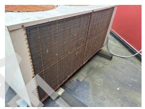
**Photo 154:** Typical condition of hail guards for condensing units. Note age and surface corrosion.
