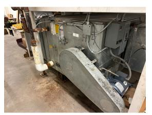
**Photo 170:** Typical AHU with heating coils only.
