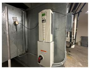
**Photo 169:** Typical VFD for interior AHU.
