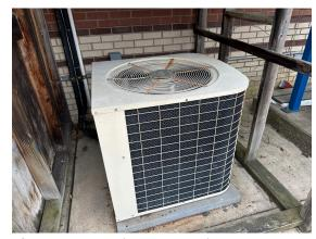
Photo 173: DX split-system condensing unit.
