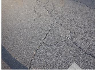
Typical allegator type cracking at the asphalt parking lot.
