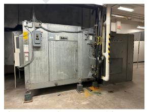
**Photo 168:** Typical Interior AHU with heating and cooling coils.
