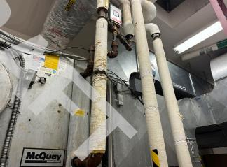
Typical condition of HHW piping, connections, and insulation.
