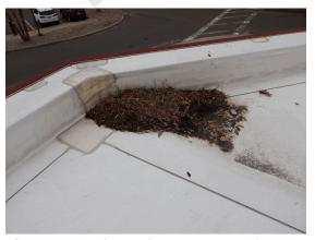
**Photo 60:** Ponding at the gym TPO membrane.
