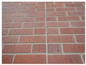
Photo 37: Elastomeric sealant.
