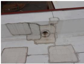
**Photo 61:** Gym: Evidence of TPO membrane repair.
