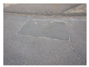
**Photo 20:** Evidence of previous repairs of asphalt vehicular pavement.
