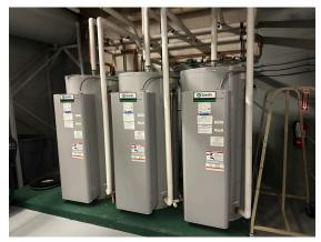
**Photo 182:** Tank-type water heaters.
