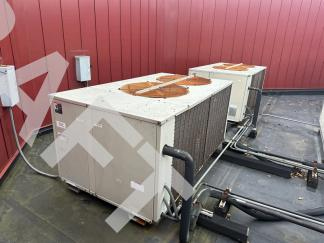
Typical roof-mounted condensing unit. Note corroded fan guards.
