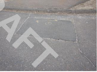
Evidence of previous repairs of asphalt vehicular pavement.
