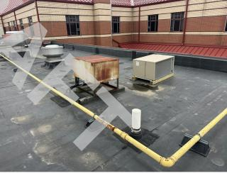
Typical roof-mounted equipment. Note surface corrosion on natural gas piping.
