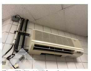
Photo 172: DX mini-split fan coil unit.
