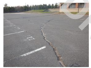
Photo 15: Linear cracking at the parking lot.
