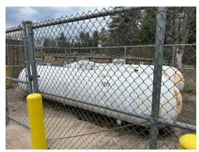
**Photo 1:** Chain link fence surrounding propane tanks for kitchen equipment.
