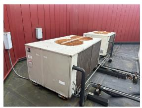
**Photo 175:** Typical roof-mounted condensing unit. Note corroded fan guards.
