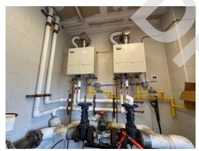
**Photo 183:** Tankless water heaters and domestic water backflow preventer.
