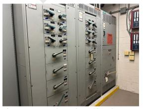
Photo 180: Main Electrical Switchboard.
