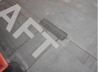
Evidence of previous repair of the EPDM roof membrane.
