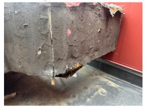
**Photo 156:** Typical condition of exterior ductwork, note deterioration of external coating/insulation.
