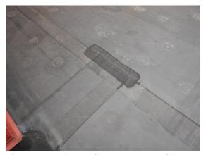
**Photo 53:** Evidence of previous repair of the EPDM roof membrane.
