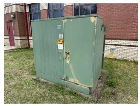
**Photo 181:** Utility owned, pad-mounted transformer.
