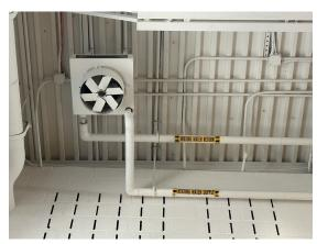
Photo 163: Typical HHW unit heater for gym.
