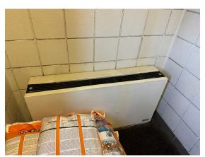
**Photo 167:** Typical HHW unit heater for stairwell.
