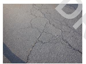
**Photo 9:** Typical allegator type cracking at the asphalt parking lot.
