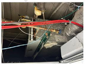
Photo 174: Typical VAV terminal units.
