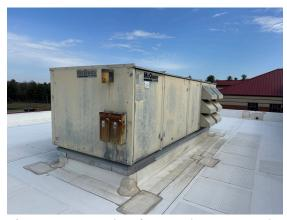
**Photo 164:** Typical roof-mounted VAV-AHU with heating only.
