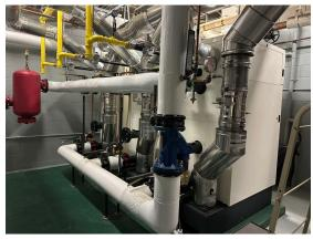
**Photo 158:** Typical condensing water boilers.
