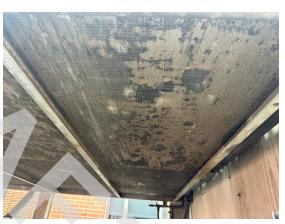
**Photo 160:** Typical condition of condensing unit fins
