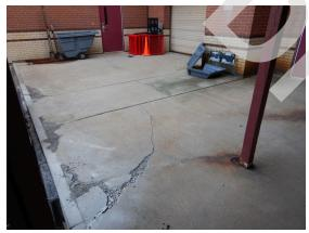
**Photo 21:** Damaged concrete pavement at the loading dock area. Typical of concrete pavement damage throughout.
