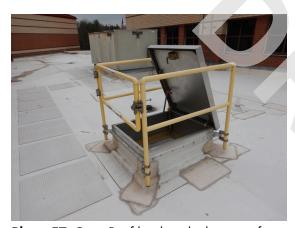
**Photo 57:** Gym: Roof hatch to the lower roof.
