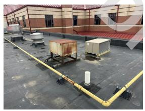
**Photo 159:** Typical roof-mounted equipment. Note surface corrosion on natural gas piping.
