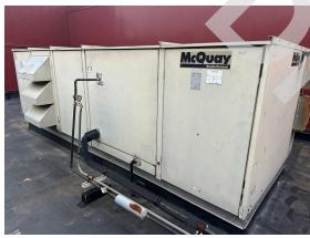
**Photo 177:** Typical roof-mounted AHU with heating and cooling coils.
