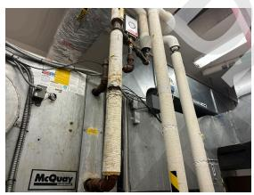
**Photo 171:** Typical condition of HHW piping, connections, and insulation.
