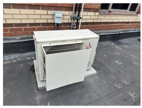
Photo 161: DX mini-split condensing unit.
