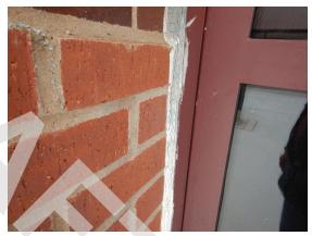
**Photo 46:** View of elastomeric sealant around the door.
