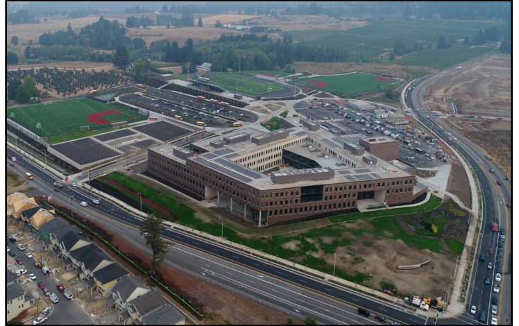
Aerial view looking northwest
