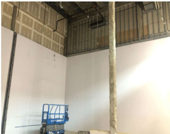
Area D, Ongoing demo of racquetball court reno.
