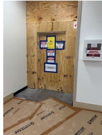
Temporary Door and Wall in Construction Area
