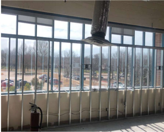
Bldg K, 2nd Floor, finished wall stud framing
