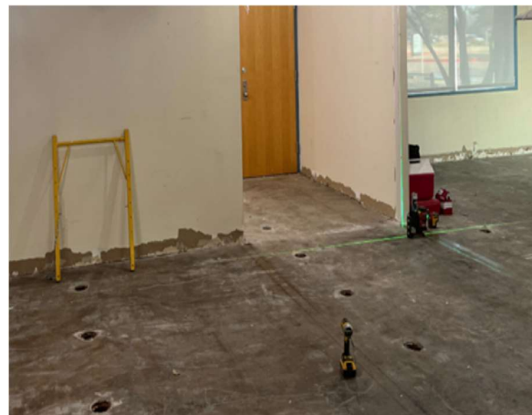
Area 1, Ongoing framing layout at Commercial Design labs
