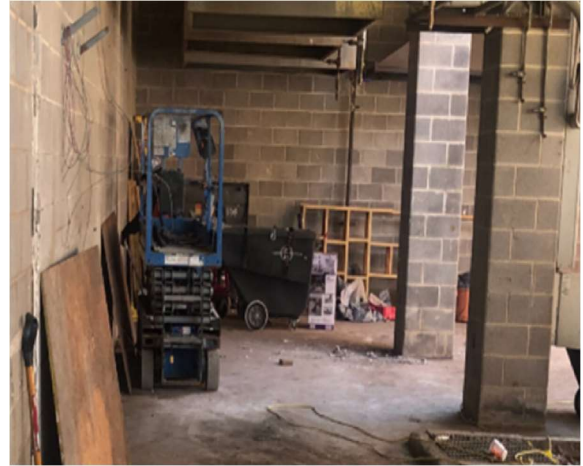
Area D, Ongoing demo of racquetball court reno.
