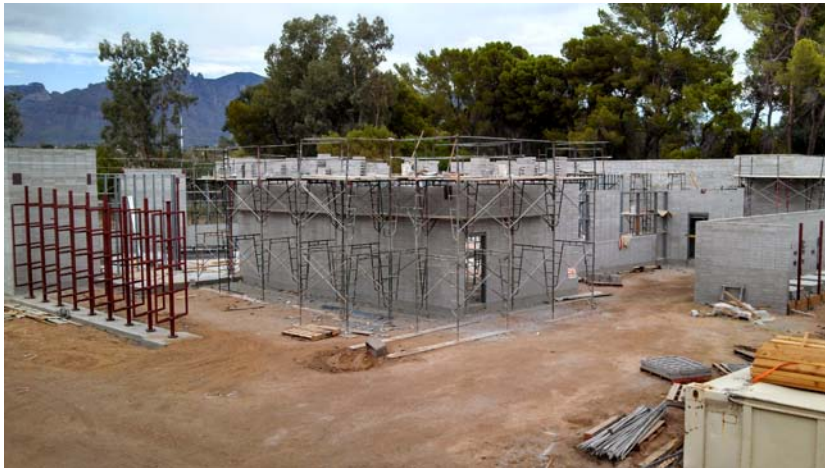
Rio Vista New Classroom Bldg. Exterior Masonry and Interior Framing
