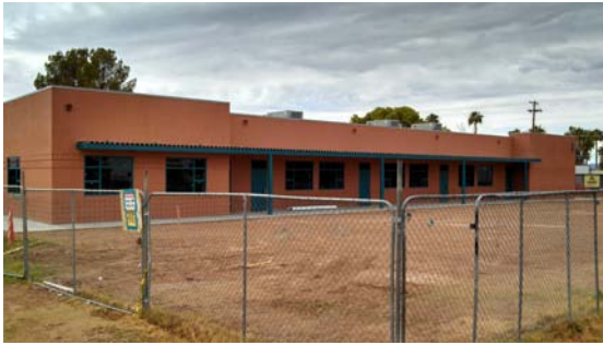
Holaway New Classroom Bldg. Exterior
