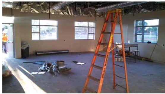
Holaway New Classroom Bldg. Interior
