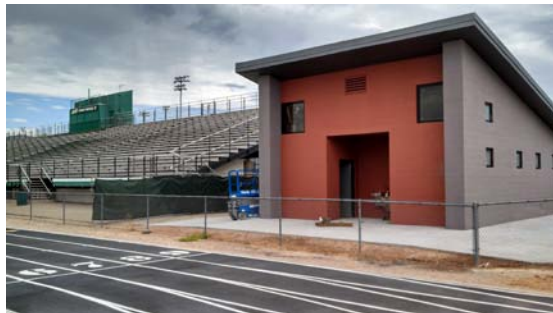
AHS New Stadium Restrooms
