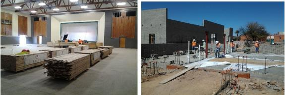
Locker Room Renovation: MP&E (mechanical, electrical, plumbing) is complete and the concrete floor is poured back. Interior framing has started.
