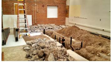
Water supply tie in for student new group restrooms by the café was completed over spring break to not disrupt campus activities. Construction of this restroom has started. All other student restrooms will be constructed or renovated during summer break.
