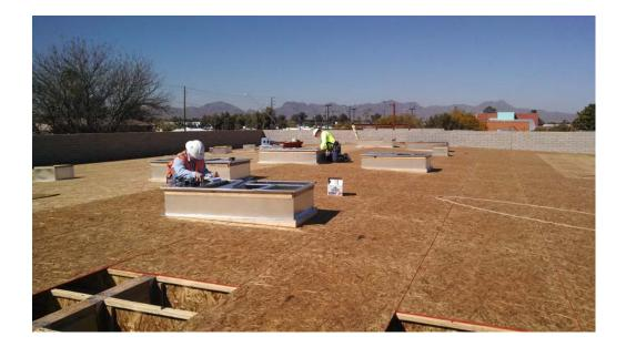
Gym Renovation: Interior finishes are being completed. The new floor is being prepped for installation. The gym lobby underground MP&E and slab on grade are complete, exterior masonry walls are being completed, and roof framing will be starting.
