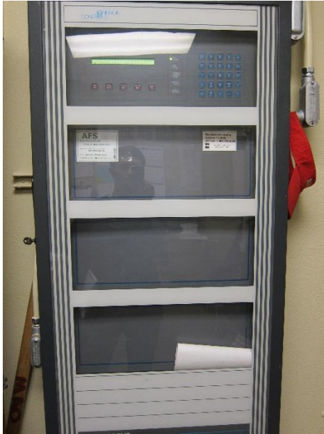
Photo E8 – Fire Alarm Control Panel
