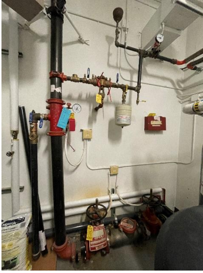
Photo M17– Fire Protection Sprinkler Riser
