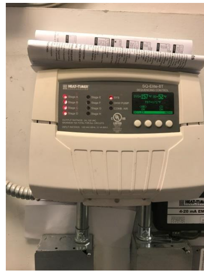
Photo M12 – Boiler Control Panel
