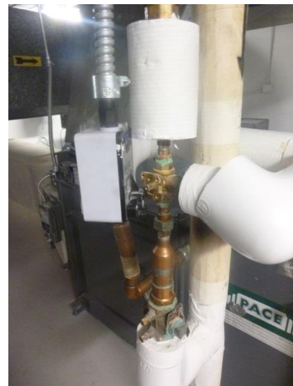
Photo M14 – AHU-1 Disconnected Control Actuator
