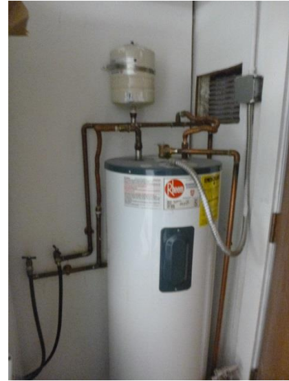
Photo M2 – Electric Water Heater
