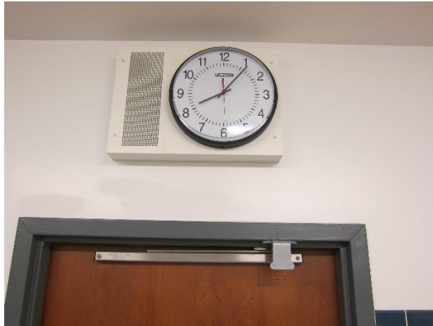
Photo E10 – Typical Combo Clock/Speaker
