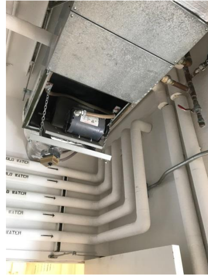
Photo M2 – Common Area Make-up Air Unit
