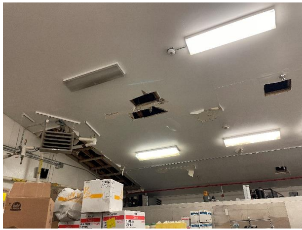
Photo M15 – Kitchen Storage Ceiling Leak Damage
