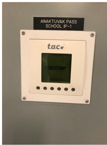
Photo M11 – Heat Recovery Control Panel
