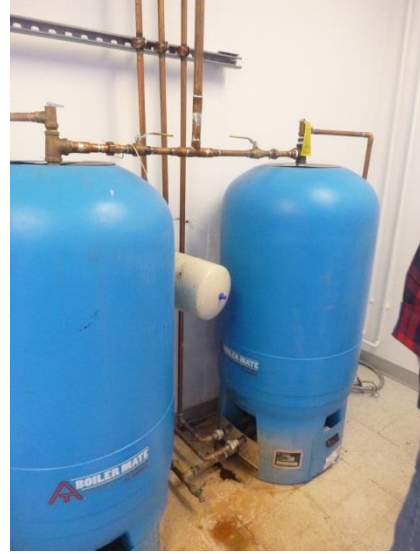
Photo M2 – Hot Water Generators
