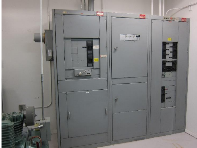
Photo E1 – Service Entrance Switchgear
