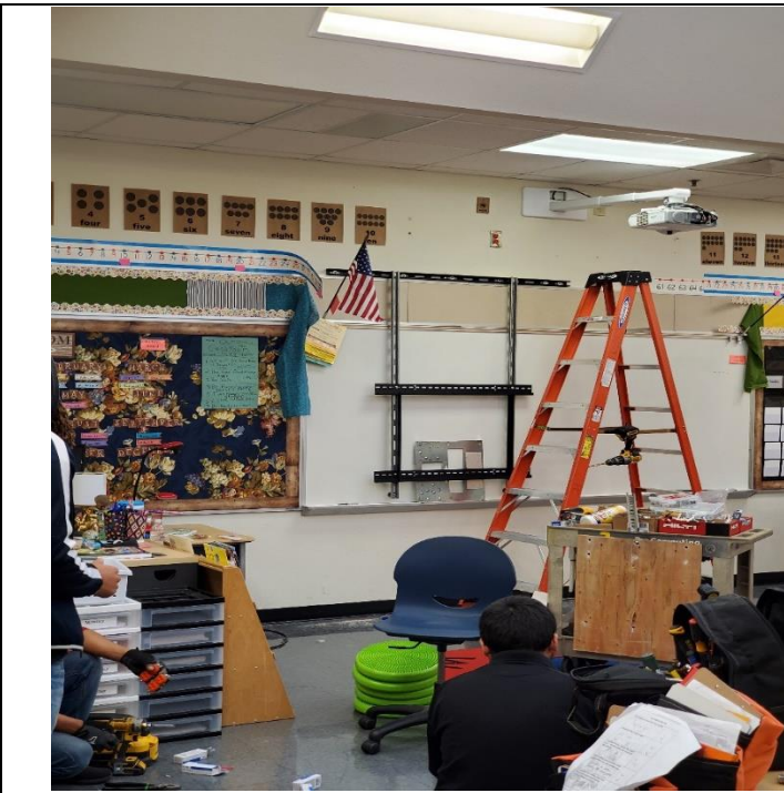
The wall mounts are manually adjustable allowing for height adjustments based on grade levels.
