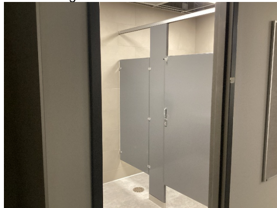
Bathroom partitions on the 2 nd floor
