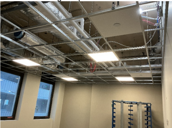
Electrical finishes on the 1 st floor
