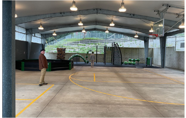
DLR Group image of Garibaldi's covered play area - one of two places to accommodate [covered] large instruction.
