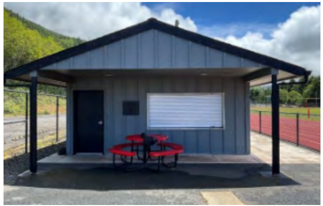
Bureau Veritas photo of Concessions & Restroom Building.
