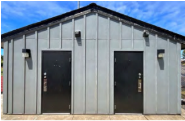
Bureau Veritas photo of Concessions & Restroom Building.
