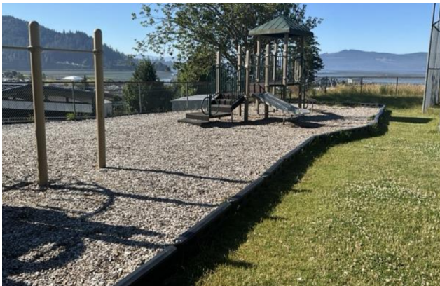
Bureau Veritas image of Garibaldi's upper playground structure.
