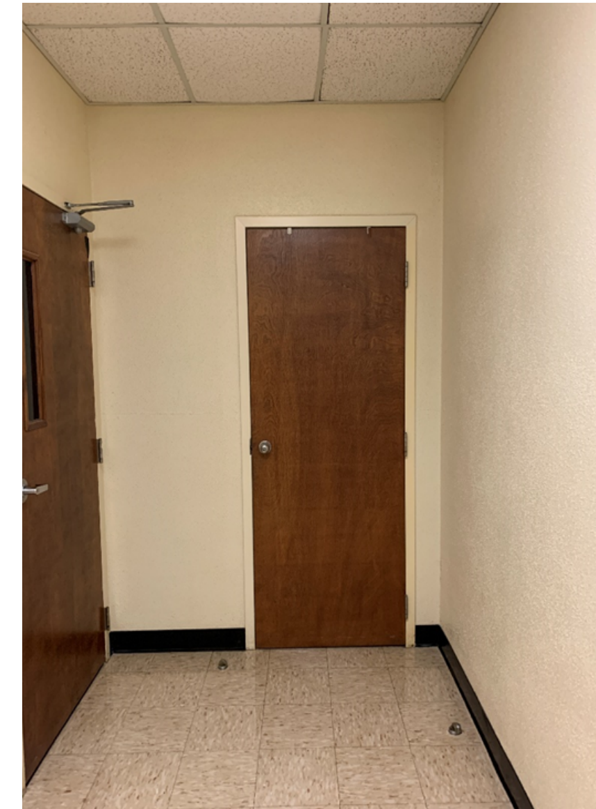
NON-COMPLIANT RESTROOMS (TAS/ADA DOORS ARE NOT FIRE RATED. NO FIRE ALARM IN THIS BUILDING.
