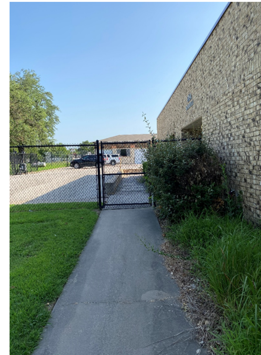
NO COVERED WALKWAY AT LIFESKILLS ENTRANCE OR MAIN ENTRANCE.
