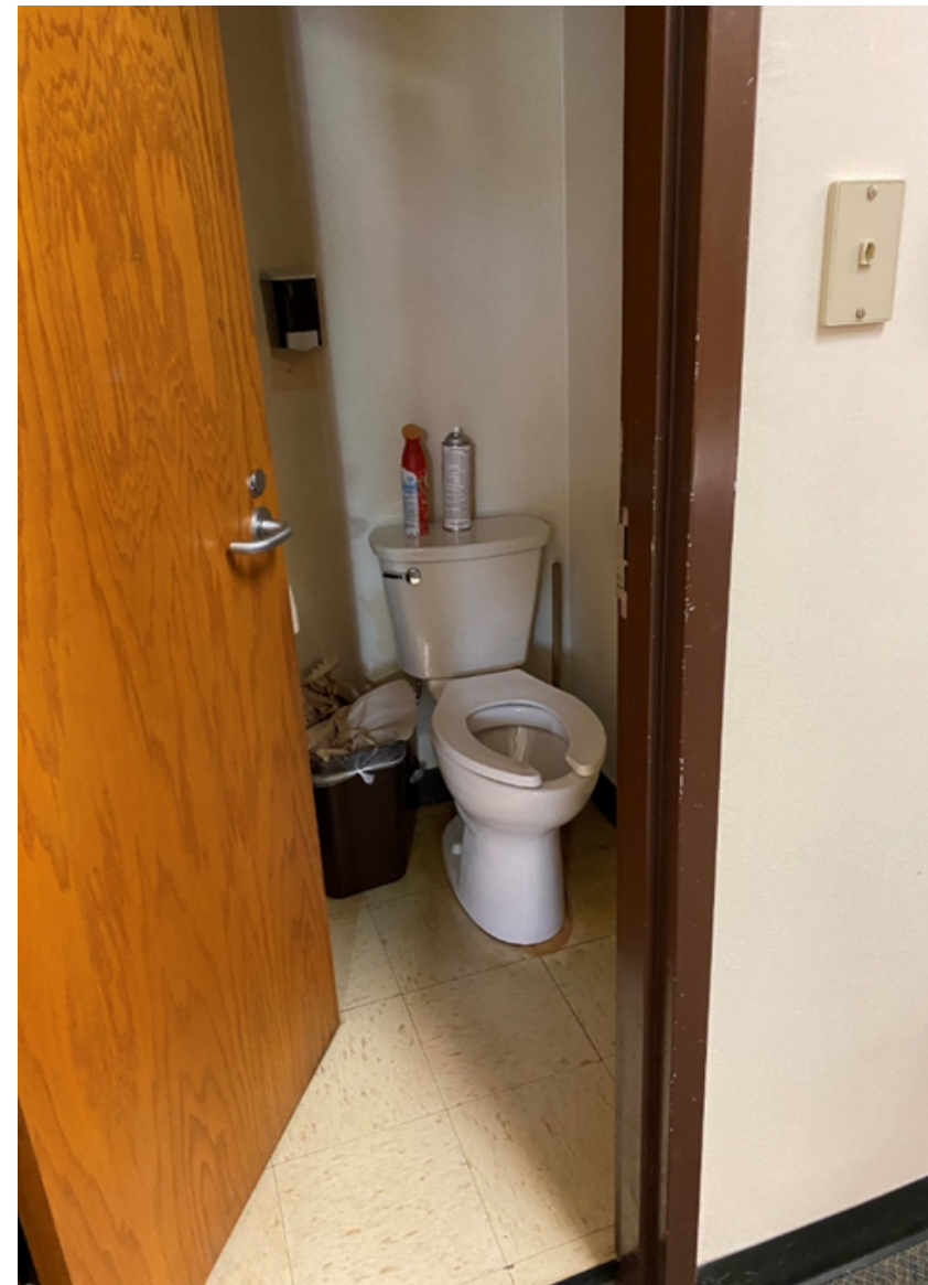
NON-COMPLIANT RESTROOMS (TAS/ADA DOORS ARE NOT FIRE RATED. NO FIRE ALARM IN THIS BUILDING.
