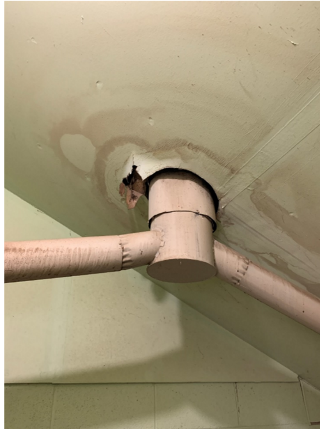
WATER PENETRATION/DAMAGE
