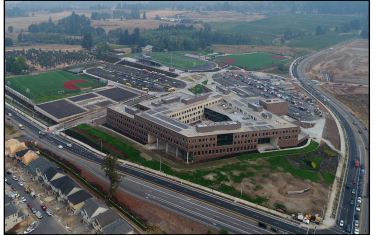
Aerial view looking northwest
