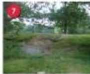
7 Revegetate Slope Drainage Area 1 Priority: High Cost: $0 Revegetate heavily eroded slope and install habitat with erosion control measures and hardy understory plants.
