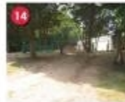
14 Establish Gravel Gathering Area Revegetate Slopes Drainage Area 1 Priority: High Cost: $0 Install gravel gravel gathering / vehicle exit area of top level catch basin. Form slope with erosion prevention measures. Provide shrubs for erosion control, habitat and understory plants.
