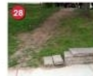
28 Revegetate Slope / New Walk & Stairs Drainage Area 5 Priority: High Cost: $0 Revegetate slope with erosion prevention and habitat plants to gain better hold. Provide shrubs for erosion control, habitat and understory plants. Consider addition of concrete walk from existing walkway to stairs.
