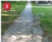
2 Biofiltration Swales Drainage Area 1 Priority: Med/High Cost: $ Create biofiltration swales along outer side of existing parking decks. Receive with slope designed.
