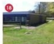
18 Rain Garden Drainage Area 2 & 2 Priority: High Cost: $0 Convert lawn area of "U" wing to rain garden. Install grade retention structure near building. Make inlet of catch basin and convert to down flow structure to remove for fully. A.K.A. Retain.
