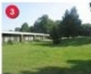
3 Rain Garden / Retention Basin Drainage Area 1 Priority: Low/Med Cost: $0 Convert lawn areas adjacent to wing to rain garden. Install grade retention structure near building. Make inlet of catch basin and convert to down flow structure. Use mulch in retention.
