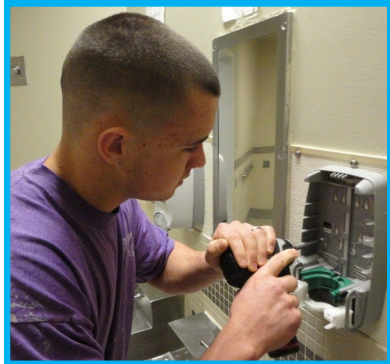
DillonM installing a soap dispenser
