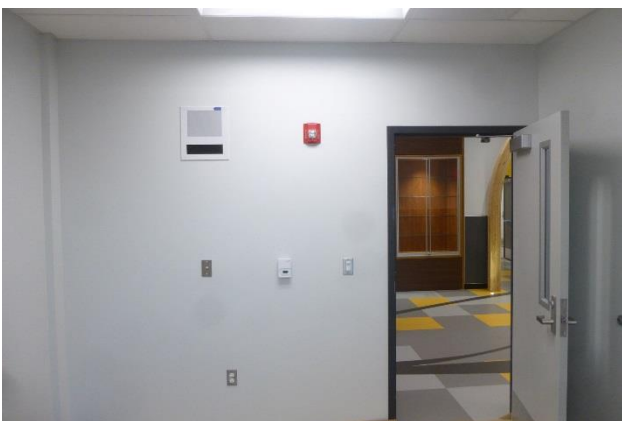
Photo E17 – New IP Speakers/Clocks & Call-Ins
