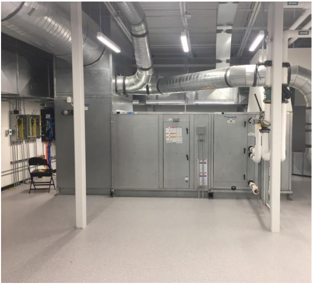
Photo M5 – Gym Addition Air Handler
