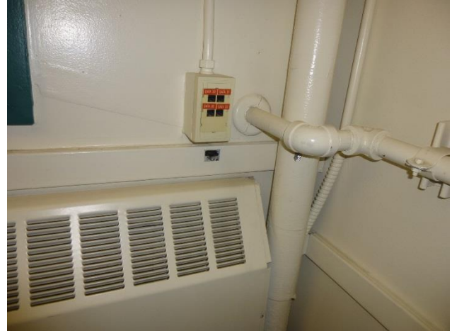
Photo E15 – Typical Older School Data Installation
