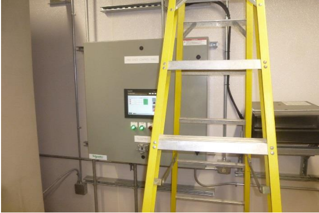
Photo E3 – Load Shed Control Panel'
