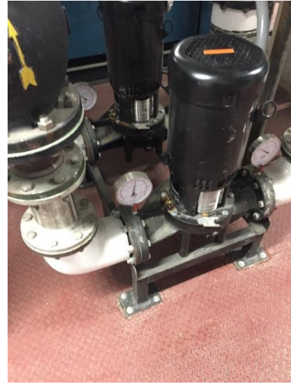
Photo M4 - Building Circulation Pumps
