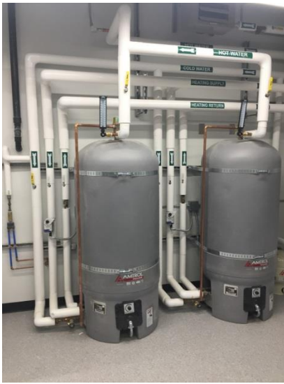
Photo M1 – Gym Addition Hot Water Generators
