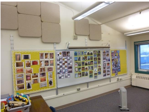
Photo E6 – Surface Raceway in Classroom
