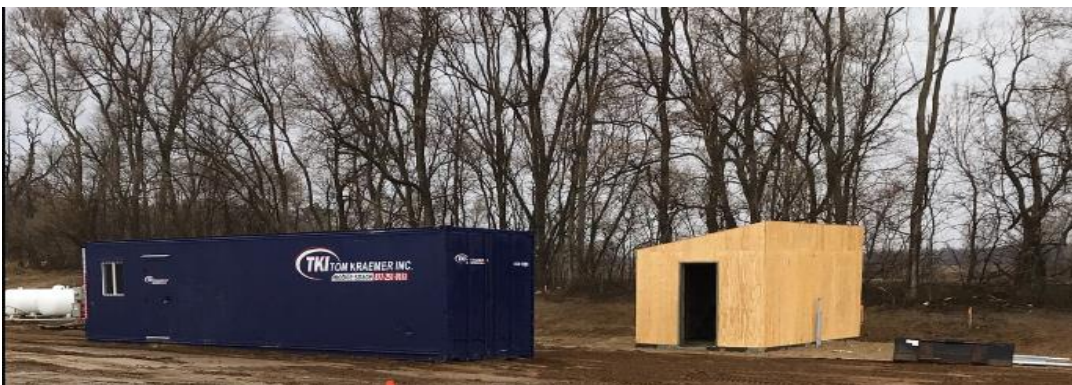
Pumphouse progress and temporary office on-site
