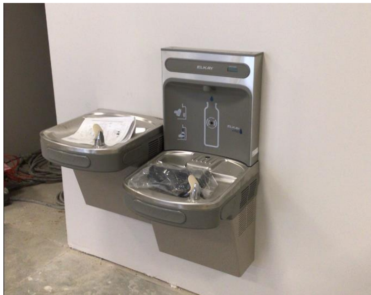
Drinking Fountain Plumbing Fixture Installation
