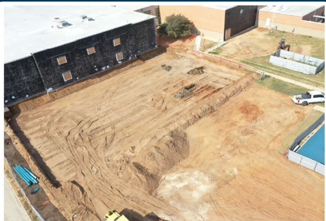
Intermediate School Building Pad Excavation
