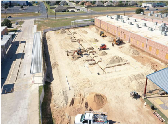
Primary School Classroom Addition (Aerial)
