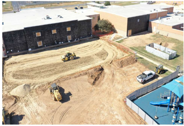
Intermediate School 2-Story Addition (Aerial)
