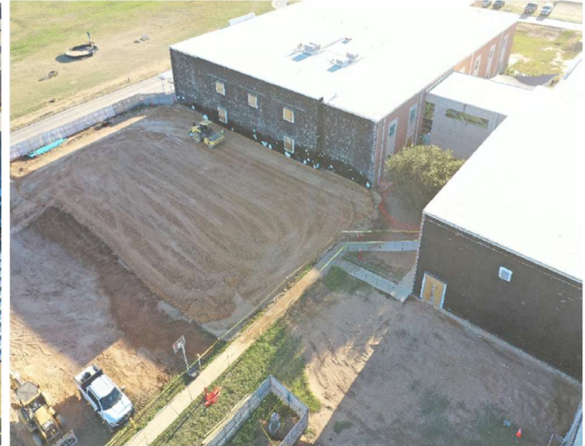
Intermediate School 2-Story Addition
