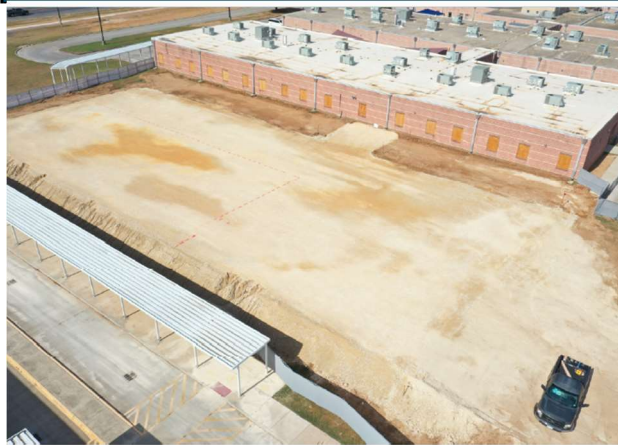
Primary School Addition Building Pad
