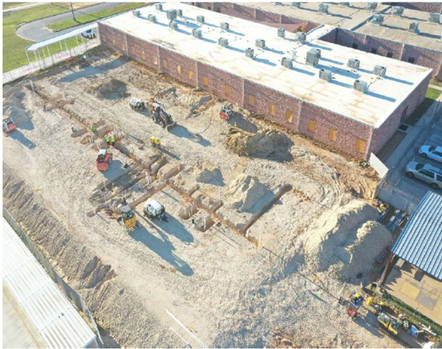
Primary School Classroom Addition
