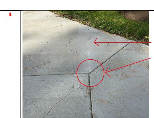
Panel has weakened concrete due to a joint that's been filled in. Replace.
