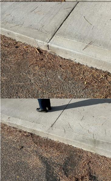
Corner of integral curb not smooth and uniform, resulting in a weakened condition.
