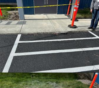
Top of concrete and top of asphalt do not meet and match. Concrete 1-2" higher then asphalt. Typical of entire west edge of parking lot.
