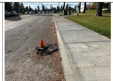
Remove excess asphalt and patch hole to be uniform and flush with existing asphalt.
