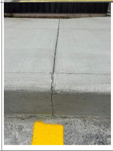
Cracks observed through curb.
