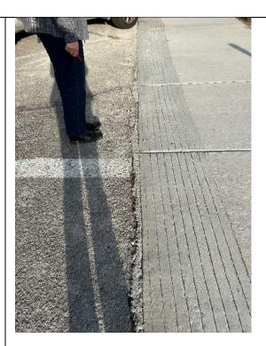
Clean sawcut line not provided. Excess concrete filling voids is not consistent with specified smooth, uniform finish and clean edges.
