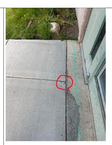
Voids and gaps in concrete finish. Repair or replace.
