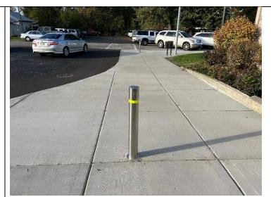
Bollard was not installed at the scored intersection as indicated, resulting in improper placement. The offset installation has weakened the concrete panel and may lead to cracking or failure. Remove and reinstall bollard at the correct scored intersection to restore structural integrity and alignment.
