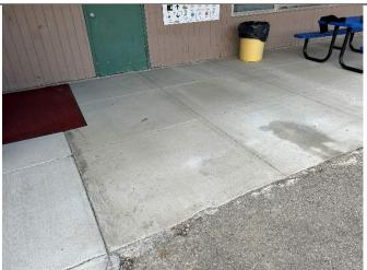
Rough patches of concrete along joints, concrete splatter, and panels with surface spalling across north side of building at playground.
