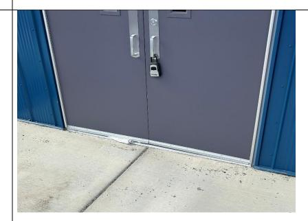
The concrete installed at the door thresholds is not acceptable. There are gaps between the concrete and the thresholds that are allowing air and rodents to enter the building.
