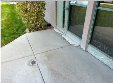
Lid is not accessible. Concrete around it is rough and poorly installed. Repair or replace.
