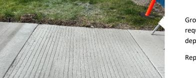
Grooves do not meet detail requirements of 3" o.c. ¼" in depth for width of ramp.
