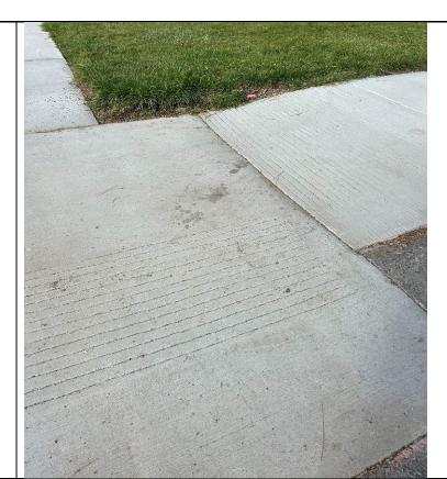
Detectable scoring not per detail. Inconsistent and lacks required depth.
