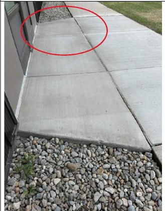
Concrete does not provide positive drainage away from doorway.
