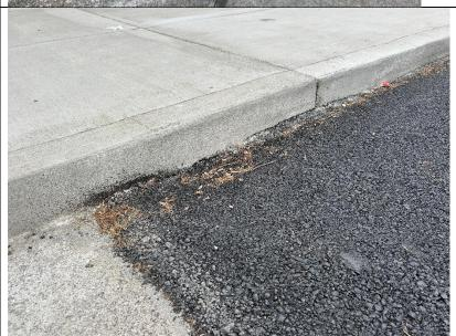
Air voids in concrete curb along base and at joint. Curb does not extend below finish grade per detail.
