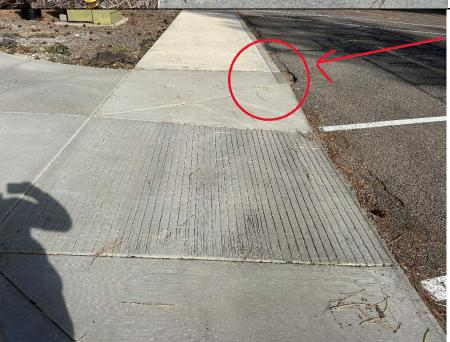
Patch back asphalt where gaps exist adjacent to concrete.
