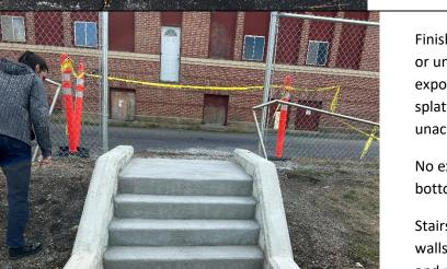
Finish on cheek walls not smooth or uniform. Chunks missing, rebar exposed on bottom corner, and splatter throughout. Finish is unacceptable.
