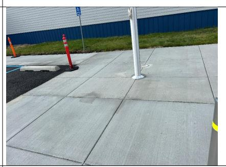
Joint finish is rough and inconsistent with specified requirements.
