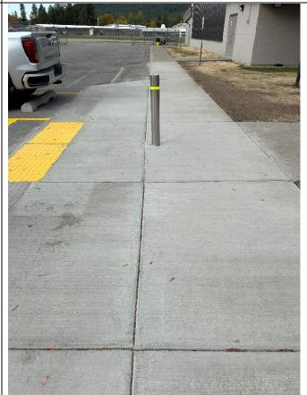
Bollard was not installed along the joint line as indicated, resulting in improper placement. The offset installation has weakened the concrete panel and may lead to cracking or failure. Remove and reinstall bollard at the correct scored intersection to restore structural integrity and alignment.
