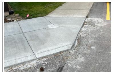
Concrete edges and splatter extend beyond curb edge.
