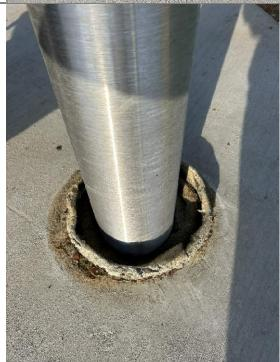
Flagpole to be installed in aluminum or galvanized sleeve. Top of sleeve to be grouted or sealed to prevent water intrusion.
