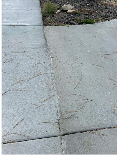
Joint finish is rough and inconsistent with specified requirements. Surface at joint is not uniform or smooth.
