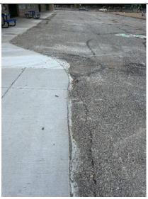
Sawcut and demolition limits do not match extents on demolition plan. Remove additional asphalt to match plans and provide clean, straight sawcut edges.
