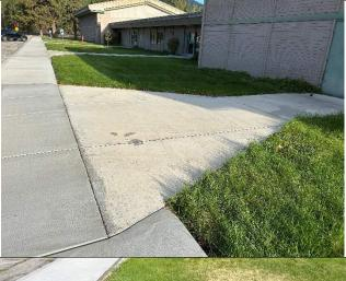
No expansion joint installed between panels.
