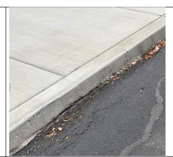
Integral curb is cracking.
