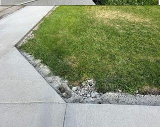
Concrete edge clean up required for entire school site. All excess concrete and forms to be removed.
