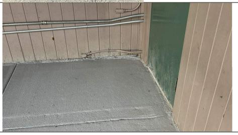
Concrete finish at building is rough and uneven, with visible tool marks and unfinished areas. Typical of entire wall under overhang.
