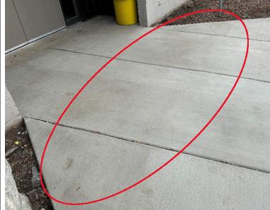
Concrete not scored per plan. A crack is observed through all four panels. Replace.
