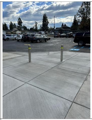
Bollards, scoring and ramp location not per plan.
