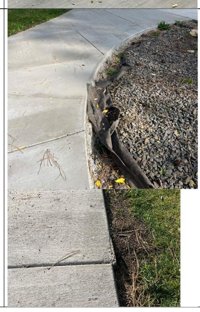
Concrete edge clean up required for entire school site. All excess concrete and forms to be removed.
