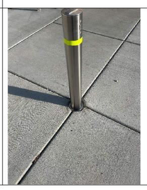
All bollards should be at concrete grade or slightly higher.
