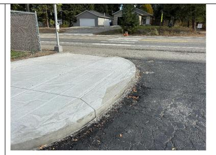
Base of concrete shows rough and uneven finish with gaps between asphalt and concrete. Voids and exposed areas present; condition not consistent with specified smooth, uniform finish and clean edges. Repair or replace.
