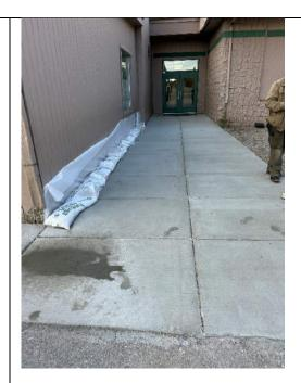
Concrete sloped into building and not per grading plan.
