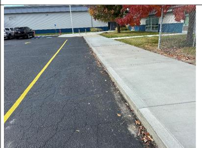
Base of concrete shows rough and uneven finish with gaps between asphalt and concrete. Voids and exposed areas present; condition not consistent with specified smooth, uniform finish and clean edges. Repair or replace.
