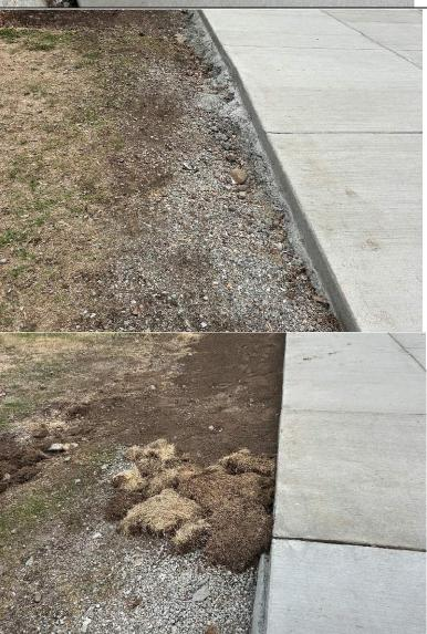
Concrete edge clean up required for entire school site. All excess concrete and forms to be removed.
