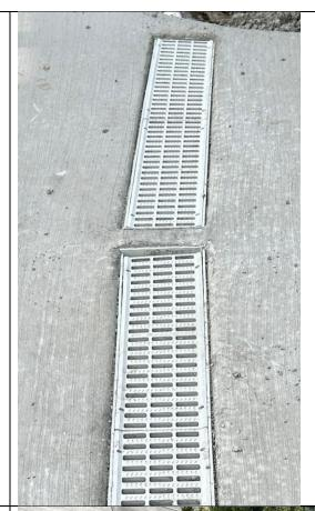
Concrete at channel drain perimeter chipped and not smooth.
