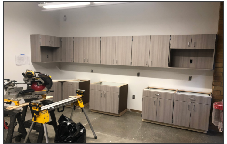
Staff lounge casework
