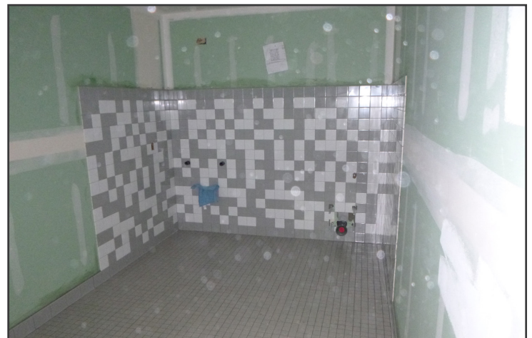
Tile work in bathrooms
