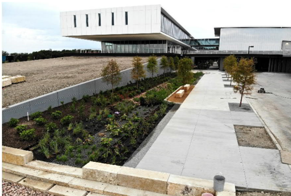
South View of Academic Building
