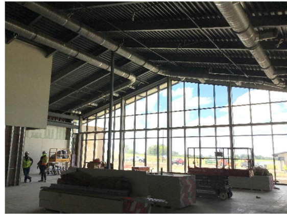
Curtain Wall at Library Area
