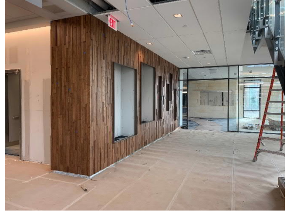
Wood Wall Installed on Level 1 of Library
