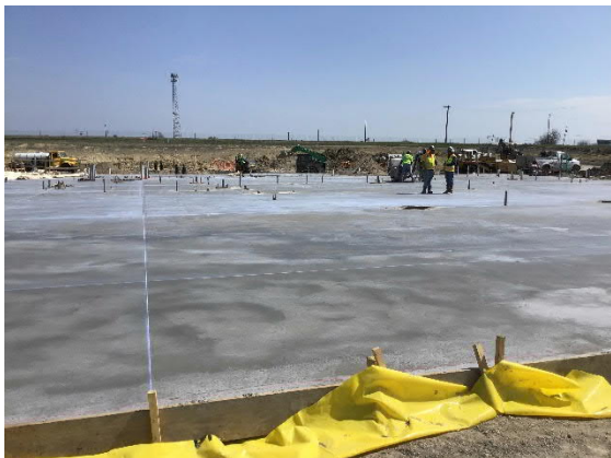
Slab Poured on Southeast Part of Building
