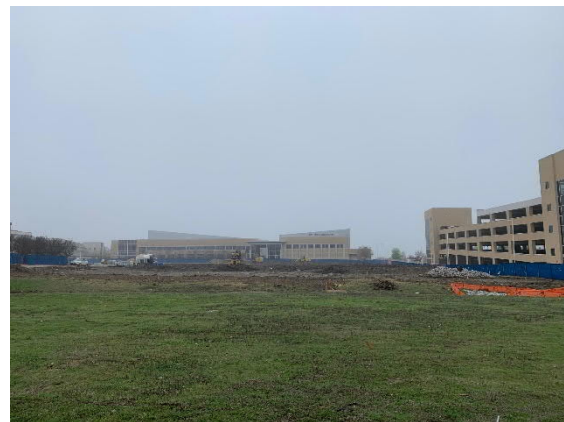
Chemical Injections Being Done at Building Pad
