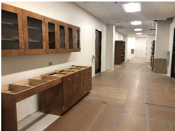
Casework Installed in Campus Commons Lab Space
