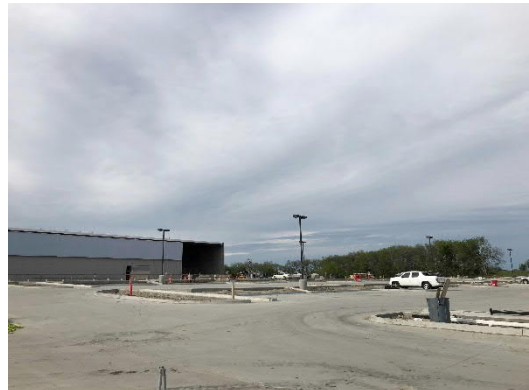
Light Poles Installed in South Parking Lot
