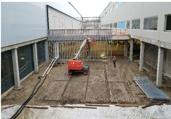
Five Star Installing Screen Wall
