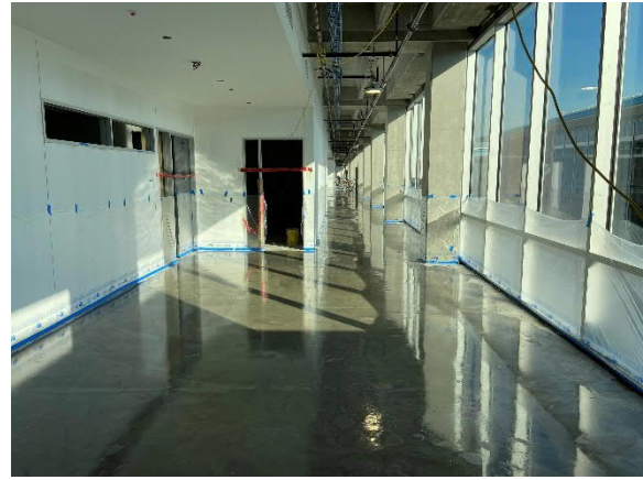
Floor Polished in Level 2 of Academic Building
